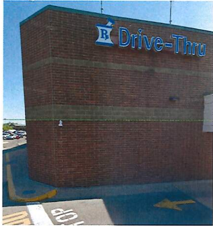
EXISTING SCOPE OF WORK: RIGHT ELEVATION - REMOVE RX DRIVE THRU AND INSTALL NEW WHITE PDT ON RACEWAY.
