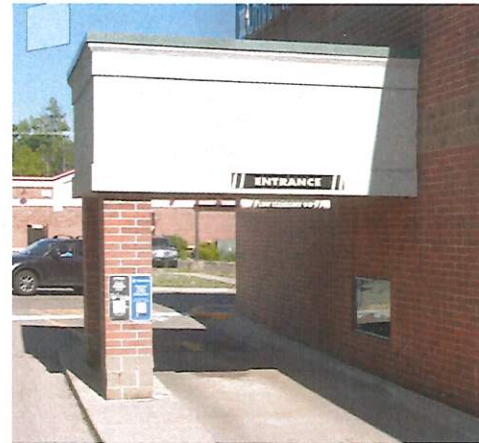
EXISTING SCOPE OF WORK: PHARMACY CANOPY - REMOVE AND INSTALL NEW EXIT LETTER SET.
