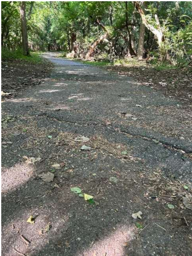
HMA Cracking
