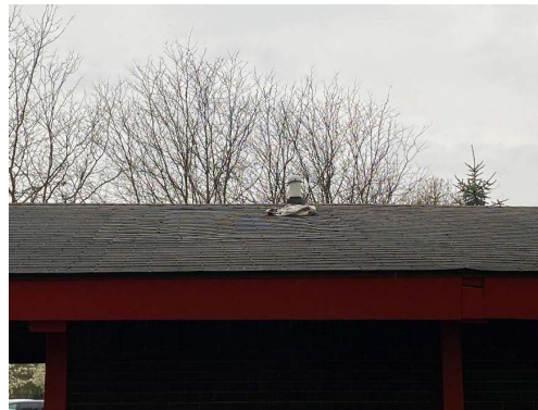
Pavilion: Peeling shingles and skylight infill translation
