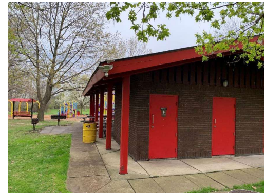
Pavilion: No gutters or downspouts present to assist with water diversion
