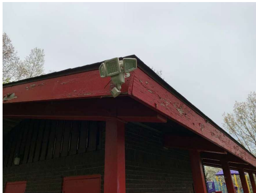
Pavilion: Facia board condition and exterior lighting
