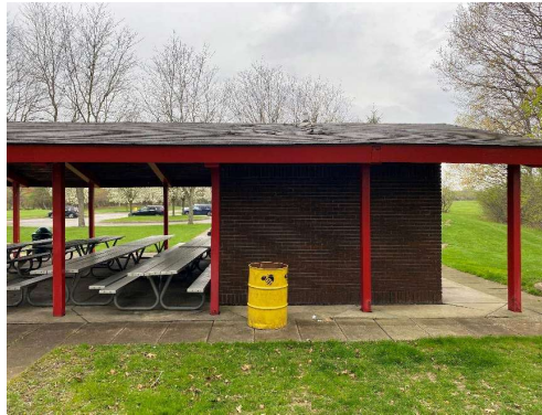
Pavilion: Covered assembly space partial and CMU wall structure
