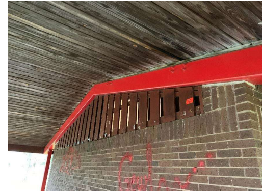
Pavilion: Worn unstained/unprotected roof decking
