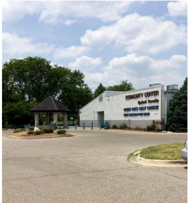
Community Center building entrance.
