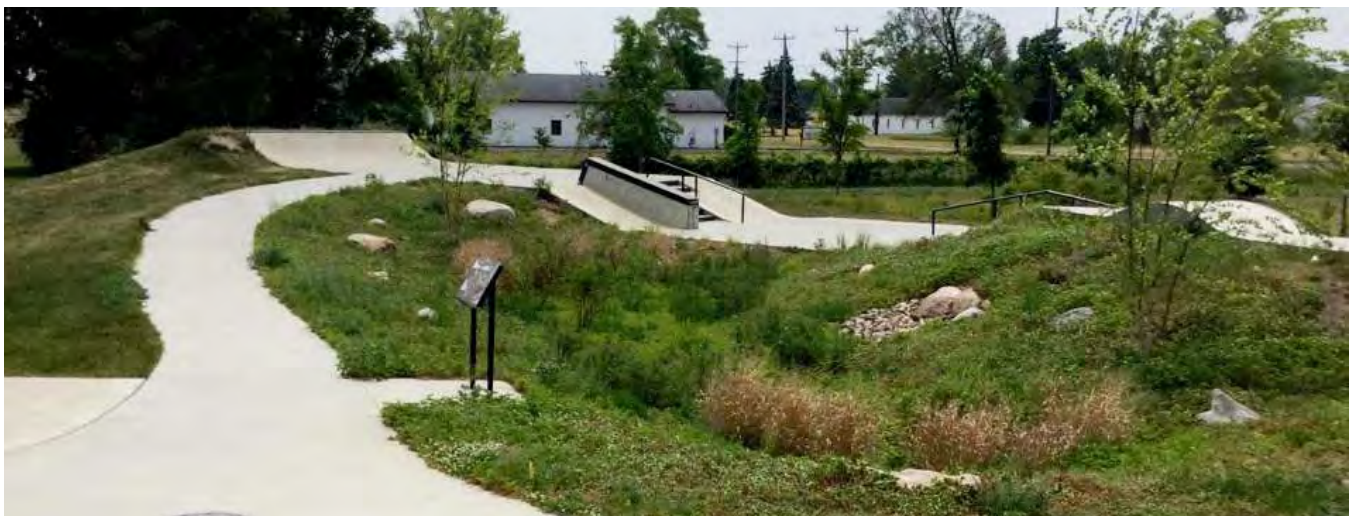
Skate park features and green infrastructure.
