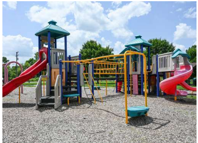
Appleridge Park play structure.
