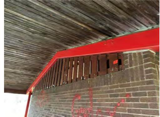
Pavilion: Worn unstained/unprotected roof decking
