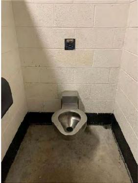
Pavilion: Clearance, dimensional and accessory requirements not met for ADA Water closet
