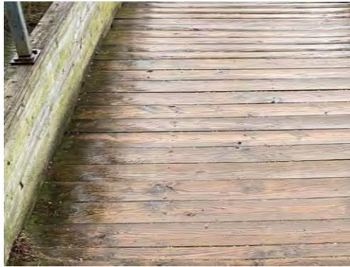
Boardwalk Bridge: B1 weathered boards with non-uniform height
