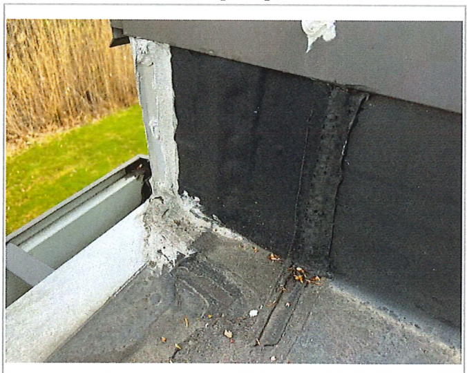
Inspect all seams repair as needed.
