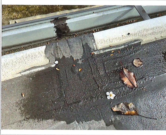
Clean prep and repair gutter edge
