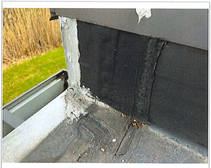
Inspect all seams repair as needed.
