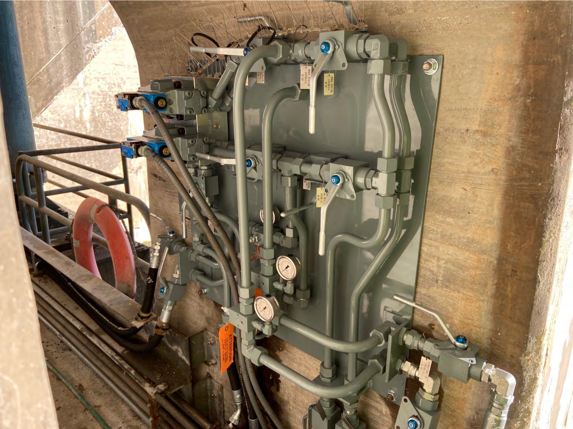
New Panel - Gates 1 & 2
