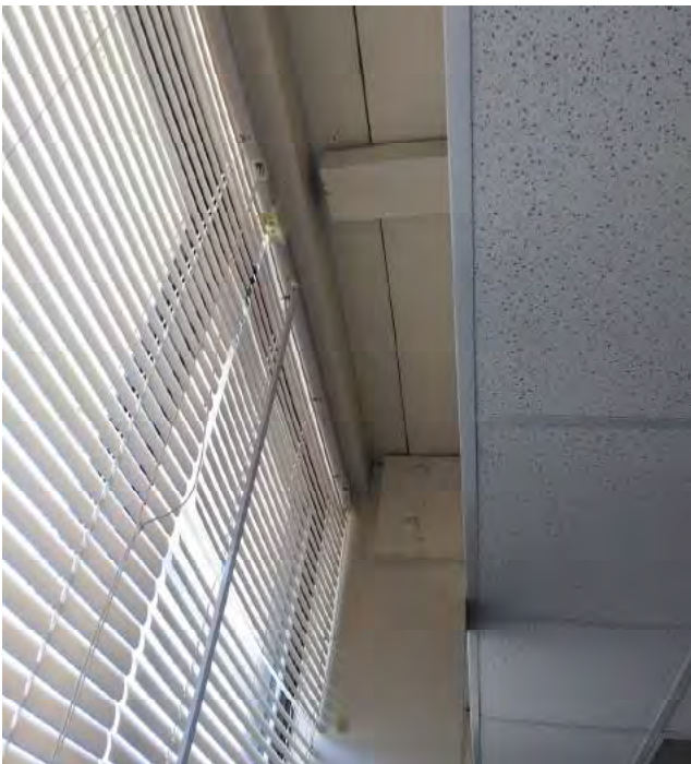
Typical window header area
