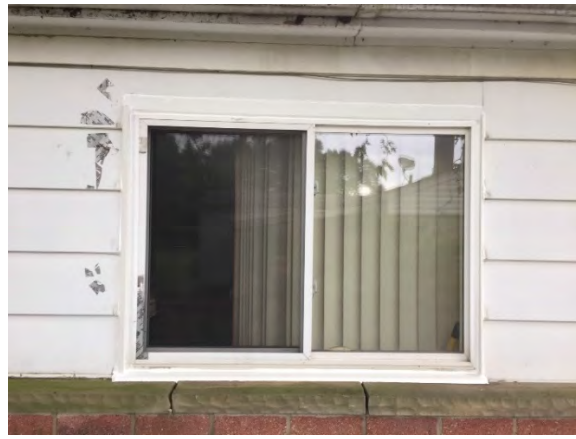
Annette's window trim after
