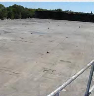
BEFORE AND AFTER SCENES OF AN EMERGENCY RESPONSE TO A CHEMICAL WAREHOUSE FIRE
