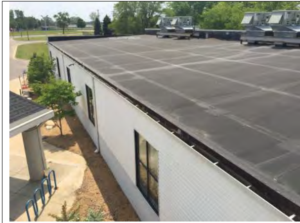
Overview – Comm. Center Section A
