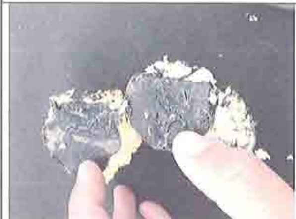
Adhesion failure between two insulation layers
