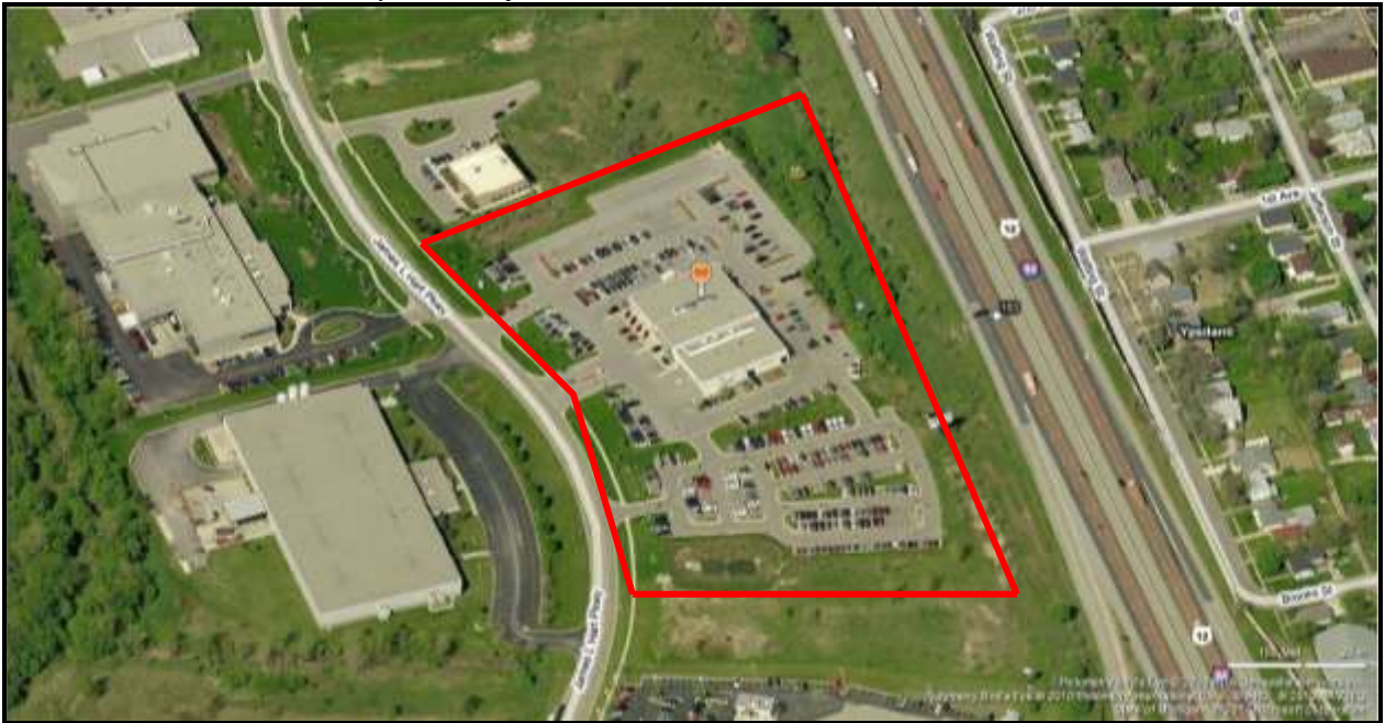
770 James L. Hart Parkway – View from the east
