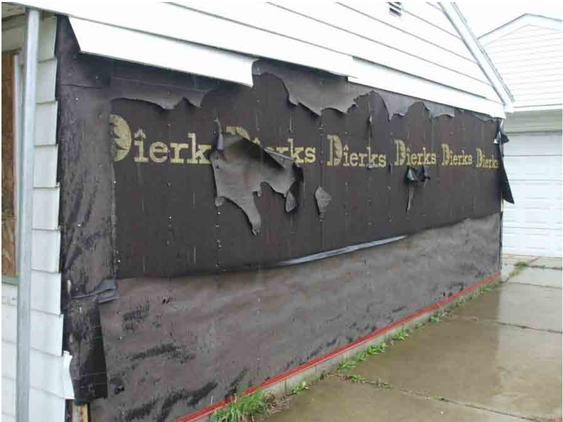
Siding removed on North side of home
