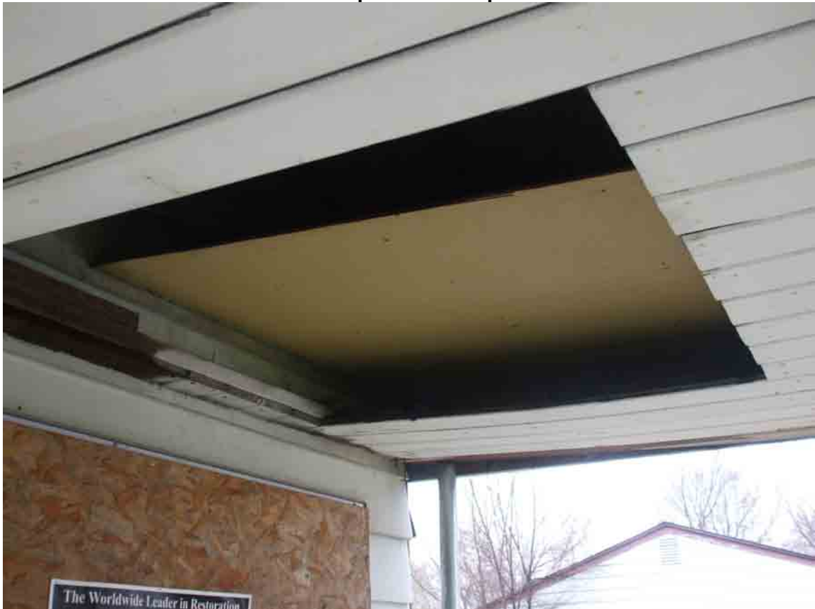
Soffit Exposed under porch
