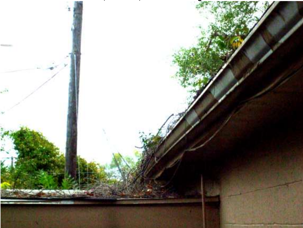
Remove leaves, branches, and debris from gutters and roof
