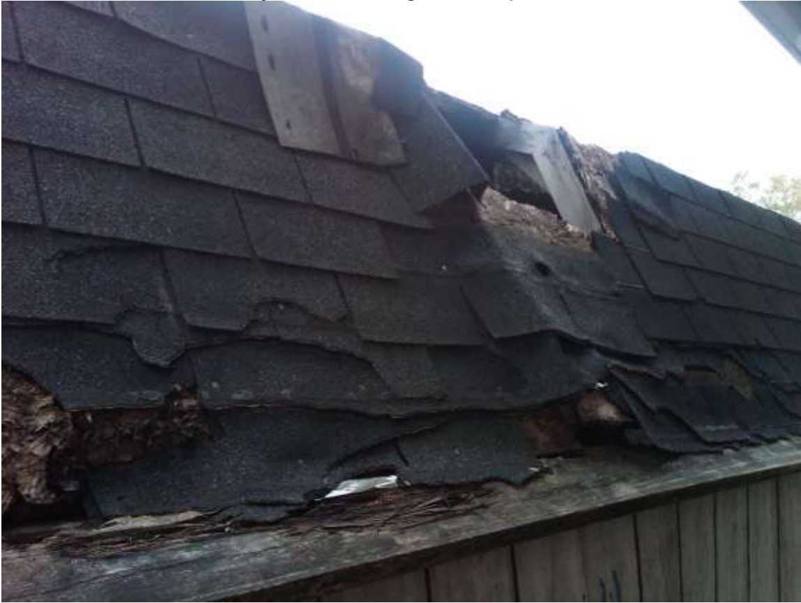
Shed adjacent to building is in disrepair/remove
