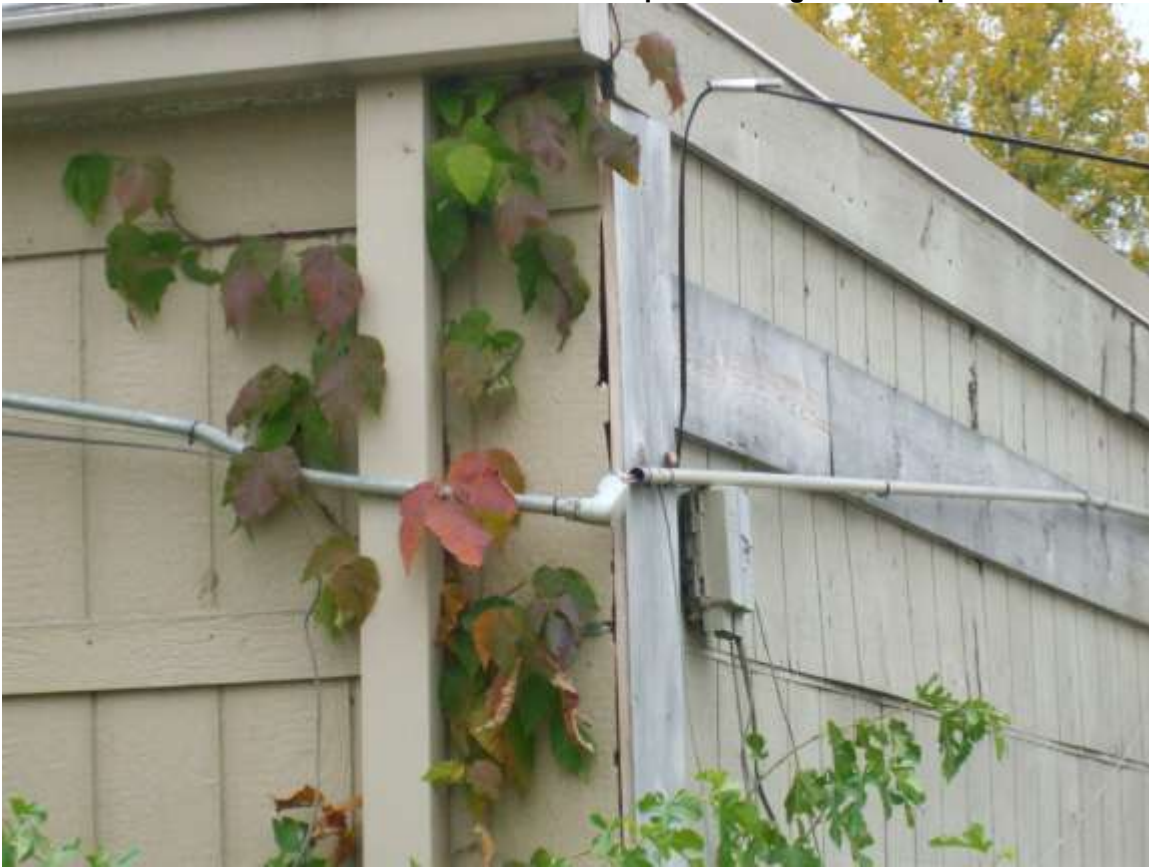
Exterior siding is in disrepair (surface defects/loose and unsecure) remove and replace
