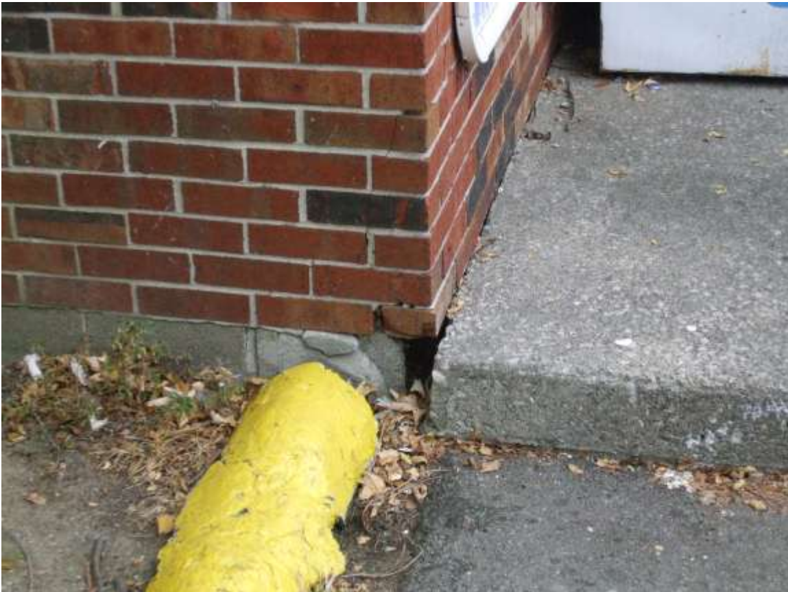
Mortar void between slab and foundation
