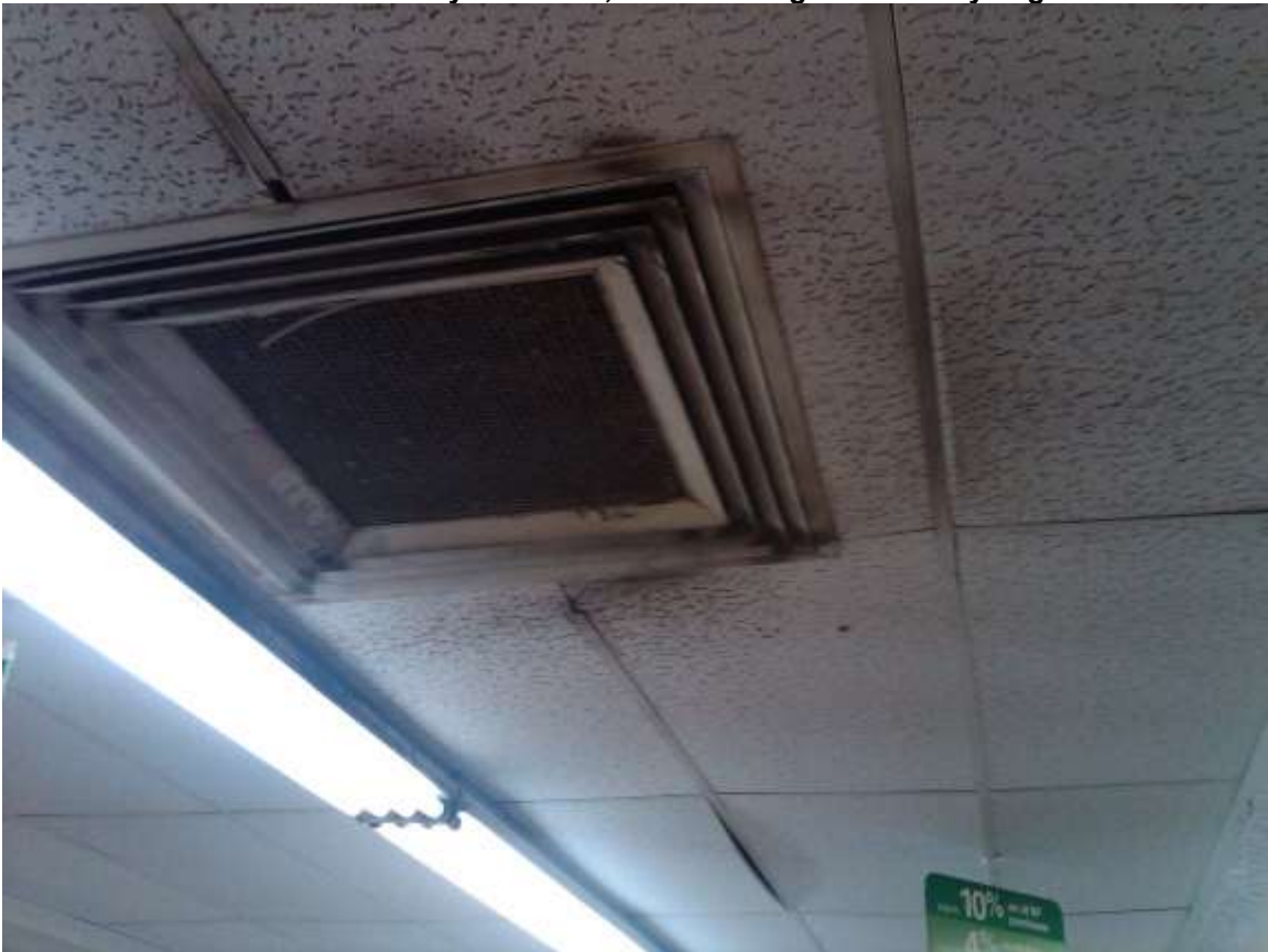
Maintain in sanitary condition, install ceiling tile securely in grid
