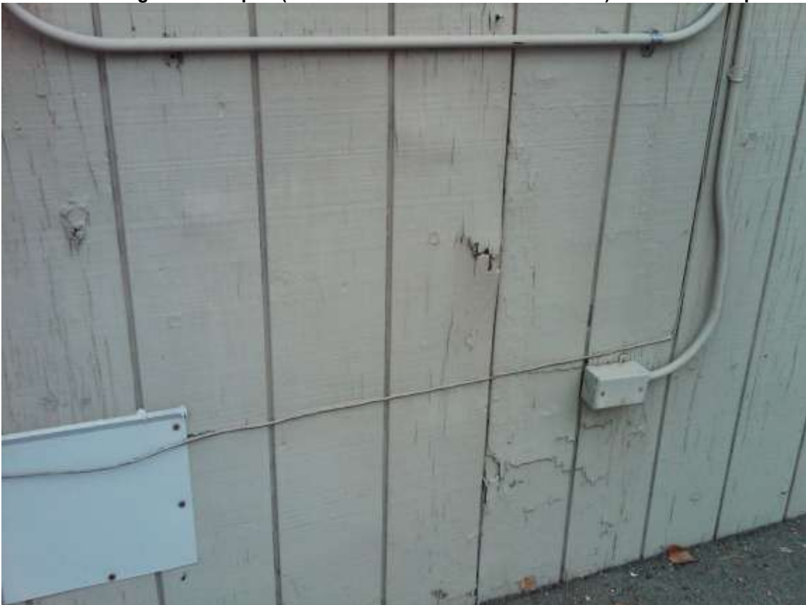
Exterior siding is in disrepair (surface defects/loose and unsecure) remove and replace
