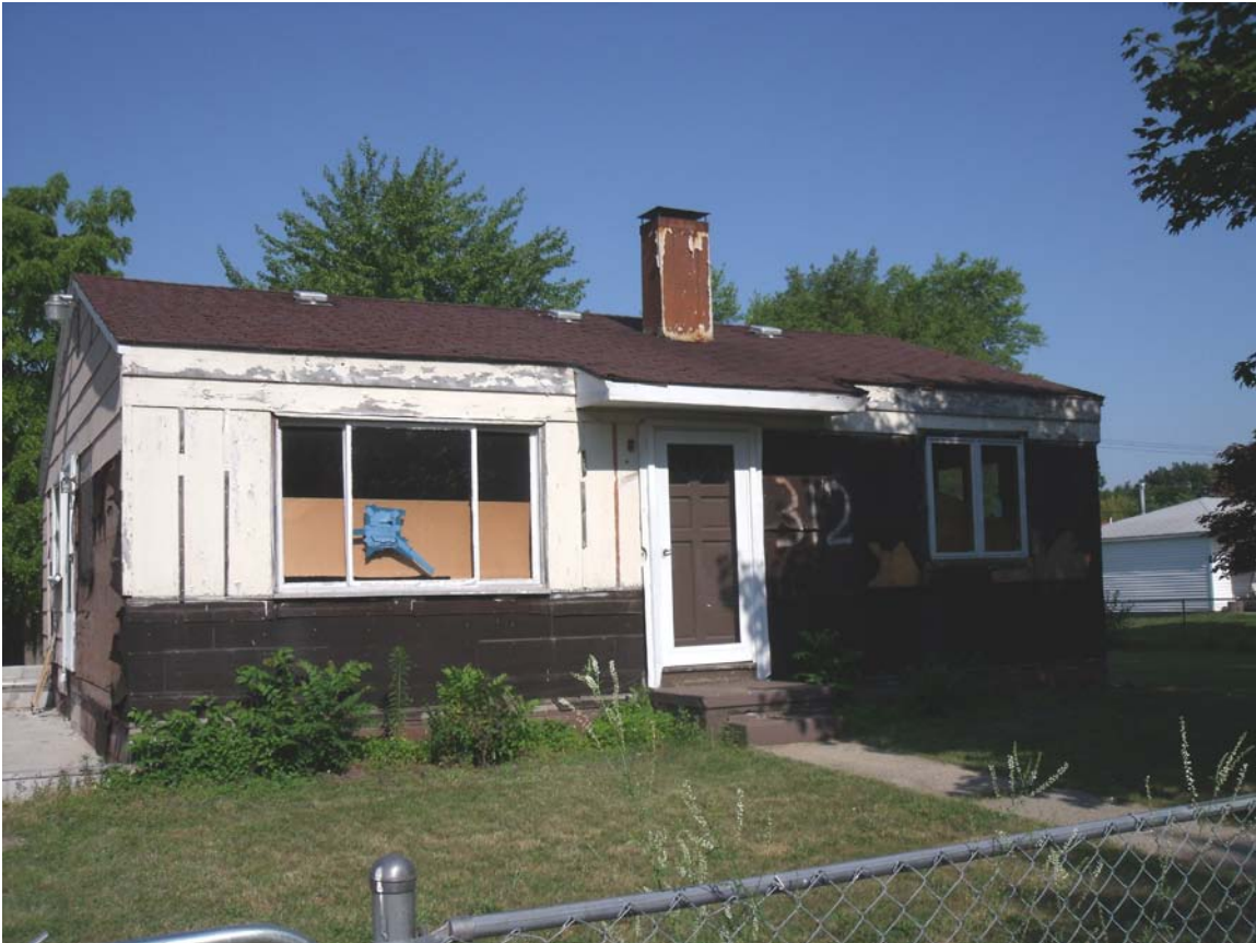
Photo #1: Exterior of home for address verification
