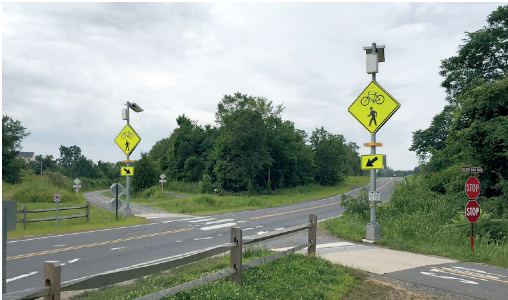
Figure 48. RRFB at a Mid-Block Crossing
