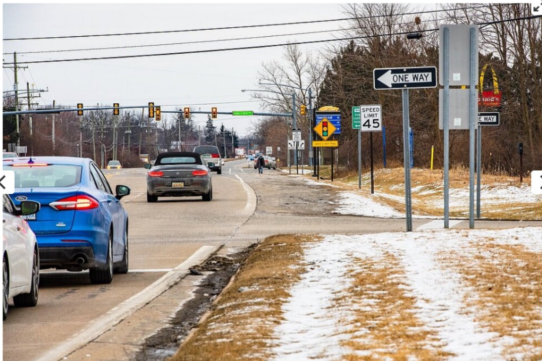
The footpath along Huron Street looking south by the eastbound I-94 exit.
