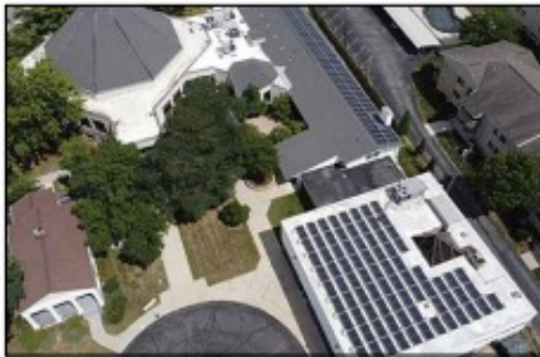
Drone photo of the Genesis campus, showing a new powerful solar installation. There are 80 panels on the flat social hall roof in the foreground and 80 panels on the south-facing slanted office roof.
