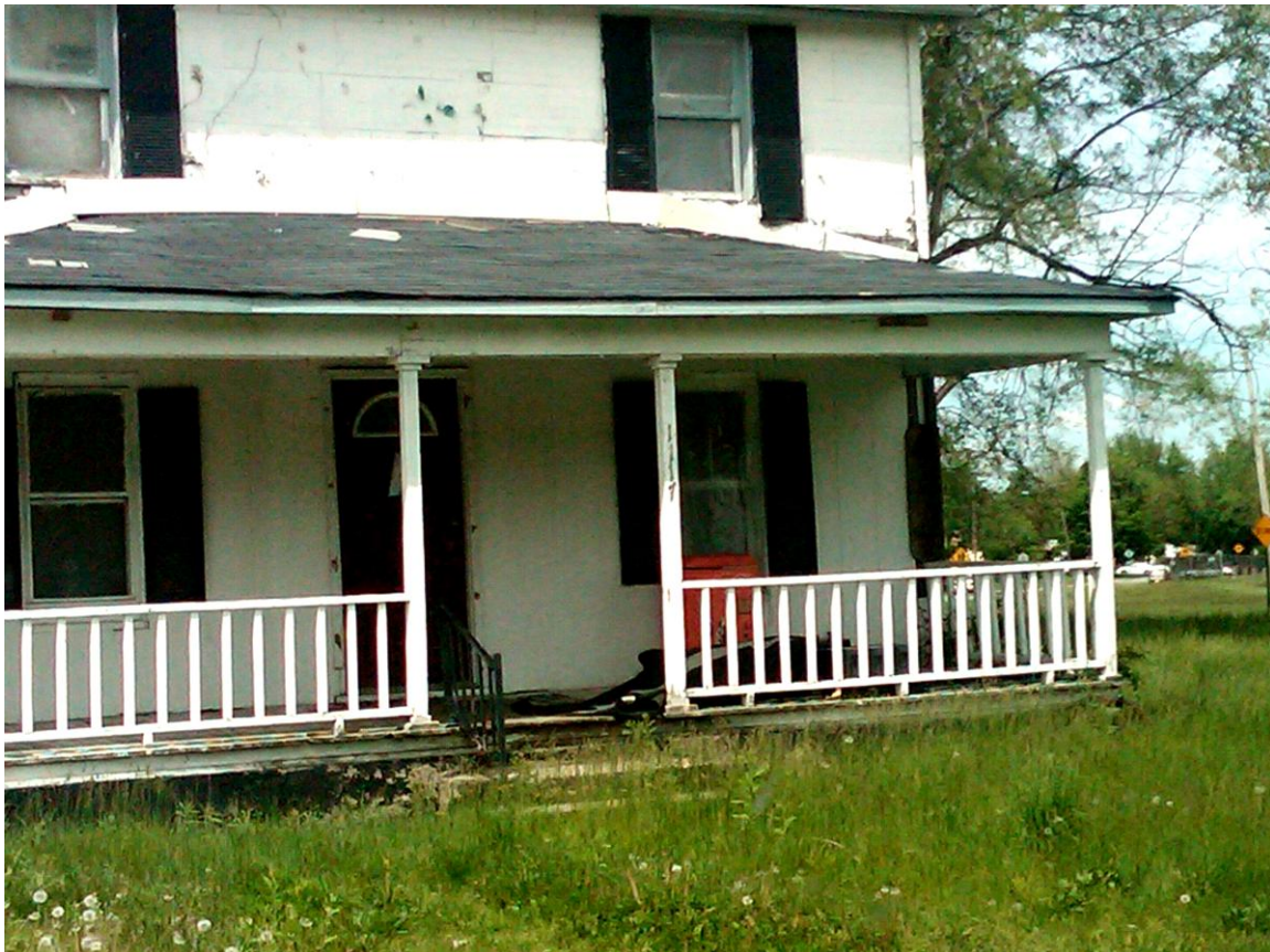
Photo #1: Exterior of home for address verification
